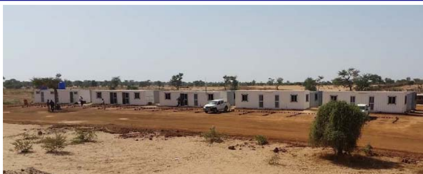
Figure 2 : Most of the infrastructure is in place
