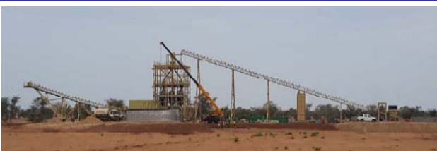
Figure 4a : Plant being constructed
